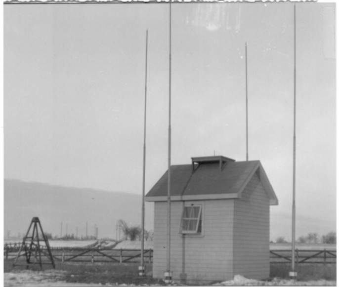
HF Direction Finding Hut
